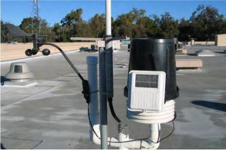
In December 2008 the GSA Grounds Department installed a weather station at the GSA Service Building located on the Government Center Campus. The wireless system sends valuable information to our Central Irrigation Computer. The weather station provides
